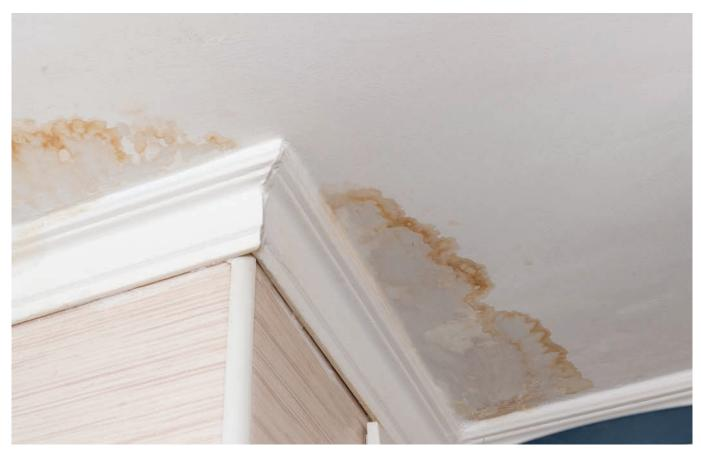
Penetrating damp will only be found on external walls, or in the case of roof leaks, on ceilings. It's caused by defects outside the home, such as missing pointing to the brickwork, cracked rendering, blocked/defective rainwater equipment, or missing roof tiles. These defects then allow rainwater to pass from the outside to the inner surfaces of your home.
