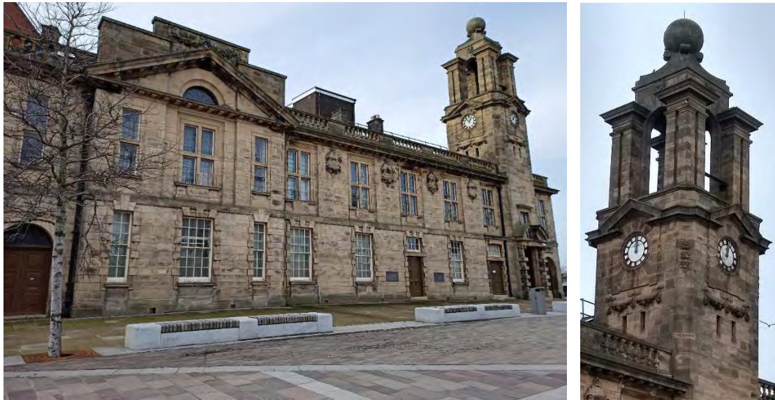
(Current views of the Magistrates Court. Source: Sunderland City Council)
