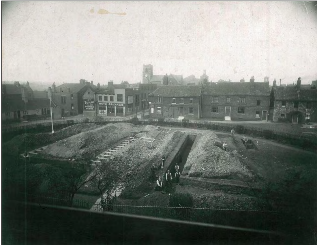
10.5: Air raid shelters being dug in the Green, 1938
