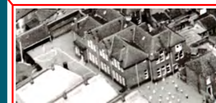
Green Terrace School was opened in 1909, replacing the Sunderland Day Industrial School. It educated the local community's children until closure in 1980, by which time urban redevelopment had resulted in most residents moving away. Demolished in 1988.
