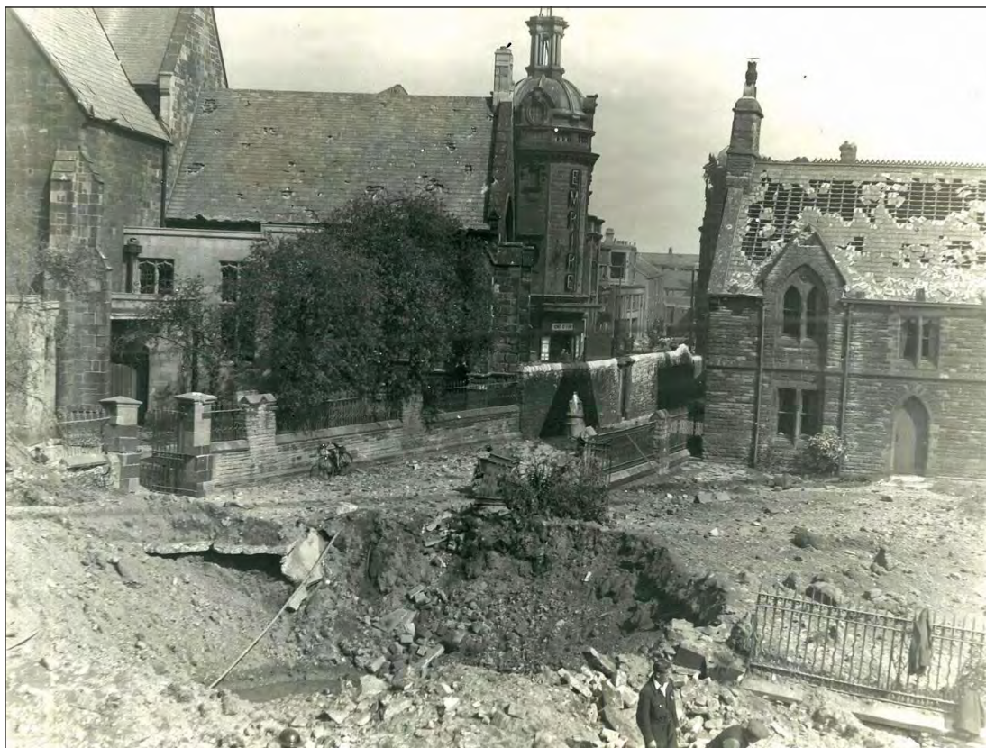
10.6: Damage caused by the bomb which struck in front of the Almshouses on Church Lane
