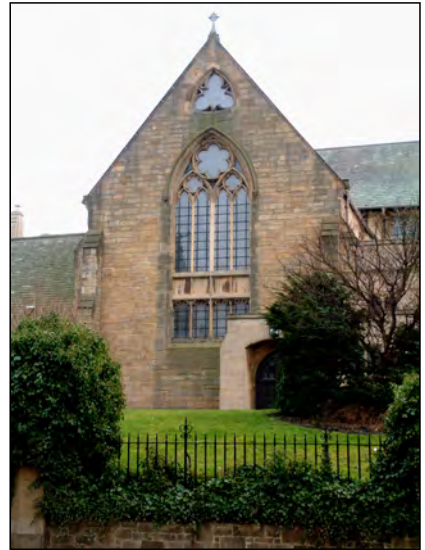
North Transept, from north
