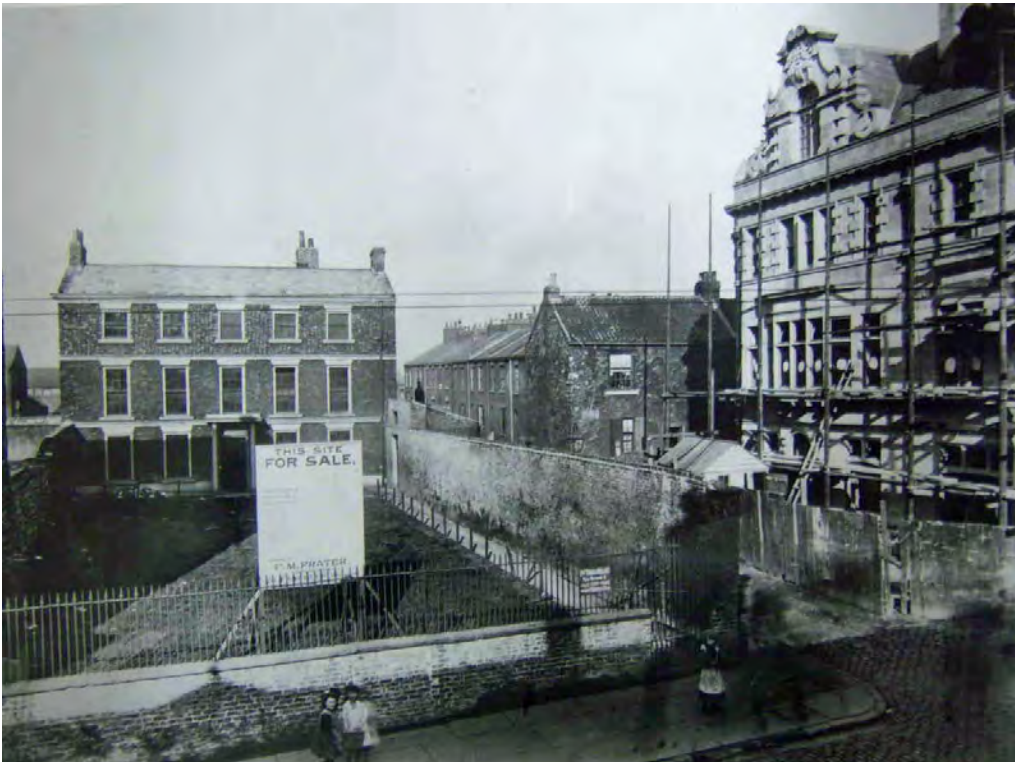
6.13: Rectory House seen shortly before demolition at the beginning of the 20th century to make way for the Empire Theatre
