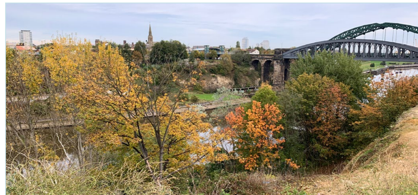
Figure 37 - View towards Monkwearmouth Railway Bridge
