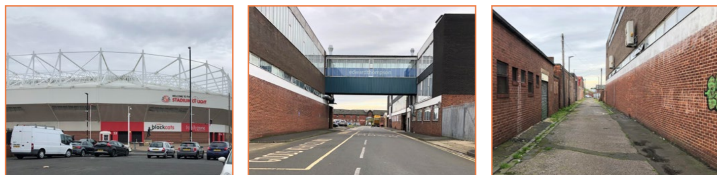
Figure 28 - Images of existing buildings on the Sheepfolds site
