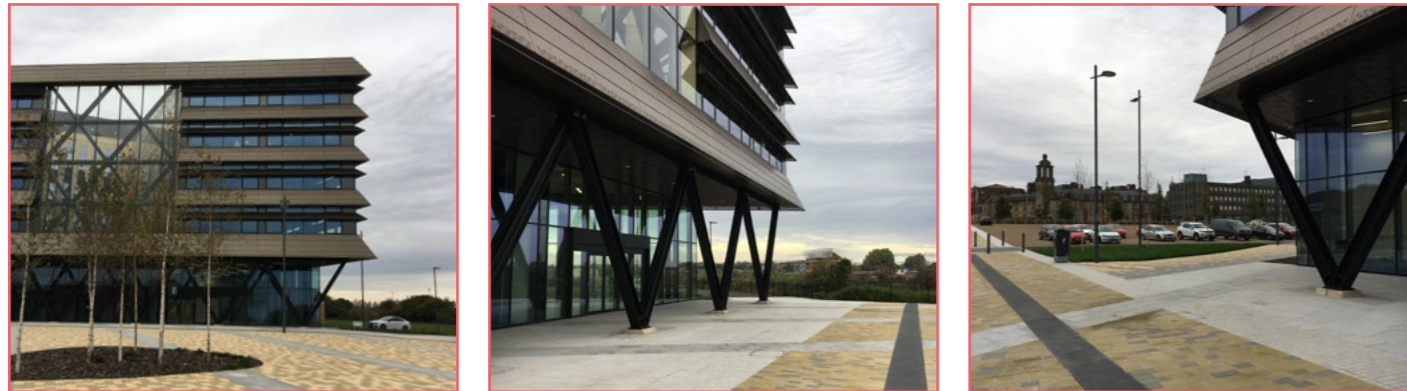
Figure 22 - Images of The Beam within The Vaux site
