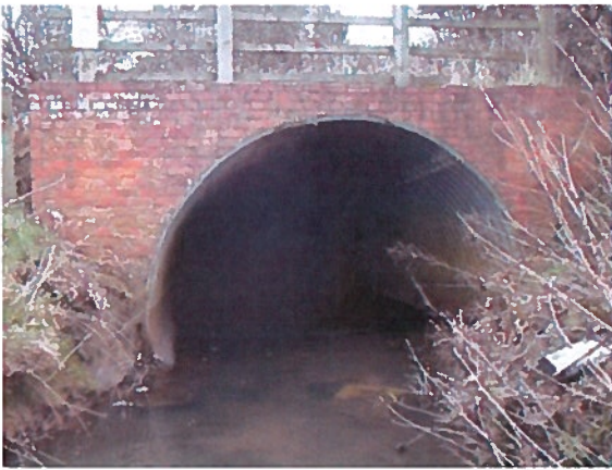
Photo 1. South-east culvert portal
