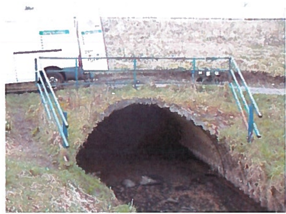
Photo 2. North-west culvert portal
