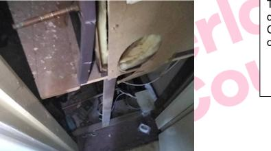
The Tank with associated debris to floor (Heating Cupboard Rm 3/005) does not contain asbestos.
