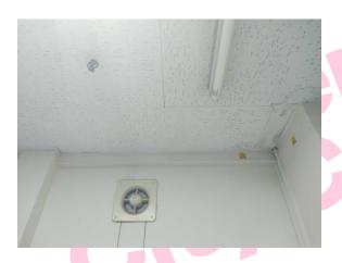
The high level horizontal boxing (insulating board) (Area: Second Floor, Room 23 Office 8) contains asbestos.
