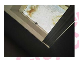
The infill panels – upstands to skylight (insulating board) (Area: Second Floor, Room 25 Finance Room 2) contains asbestos.
