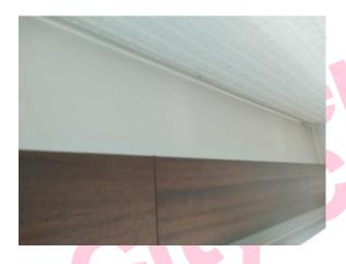
The high level horizontal boxing (insulating board) (Area: Second Floor, Room 35 Paddy Cronin Office) contains asbestos.
