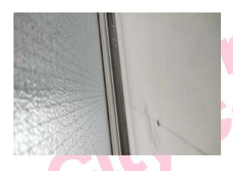
The window – fillet to window reveal behind cladded RSJ (insulating board) (Area: Second Floor, Room 48 First Aid Room) contains asbestos.
