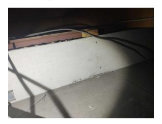
The debris to tops of ceiling tiles (insulating board) (Area: Second Floor, Room 8 Server Room) contains asbestos.
