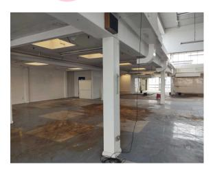
The boxing – cladding to columns (insulating board) (Area: Second Floor, Room 56 Racking Store) does not contain asbestos.
