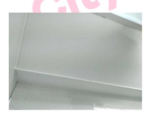
The high level horizontal boxing (insulating board) (Area: Second Floor, Room 17 Female WC and Lobby) contains asbestos.
