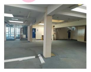
The vertical boxing over columns and RSJ's (insulating board) (Area: Second Floor, Room 26 Main Office) contains asbestos.
