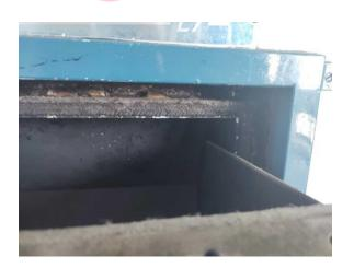
The vessels – rope seal to incinerator (textile) (Area: Second Floor, Room 51 Female WC and Lobby 2) contains asbestos.
