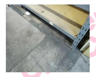
The floor (tiles & adhesive) (Area: Second Floor, Room 70 Filing Store) does not contain asbestos.
