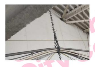
The fire breaks to tops of wall outside female wc (Area: Second Floor, Room 26a: Tank room (within ceiling void)) contains asbestos.
