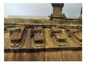
The vessels – debris to boiler (textile) (Area: Second Floor, Room 71 Boiler Room) contains asbestos.
