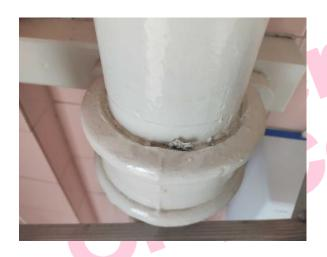
The downpipes – filling to pipe flange knuckle (insulation) (Area: Second Floor, Room 48 First Aid Room) does not contain asbestos.
