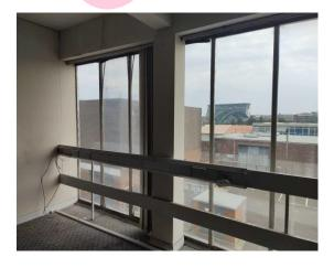
The vertical boxing (insulating board) (Area: Second Floor, Room 68 Electric Office) contains asbestos.
