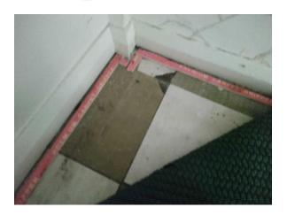
The floor (tiles & adhesive) (Area: Second Floor, Room 54 Ex Store) does not contain asbestos.
