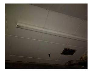
The ceiling tiles (insulating board) (Area: Second Floor, Room 71 Boiler Room) contains asbestos.
