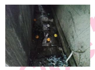
The loose lying panel behind convector heater (insulating board) (Area: Second Floor, Room 75 Main Workshop) contains asbestos.
