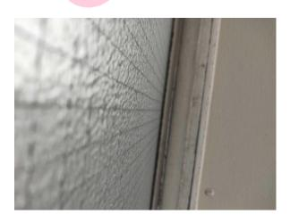
The window – fillet to window reveal behind cladded RSJ (insulating board) (Area: Second Floor, Room 47 Comms Room) contains asbestos.
