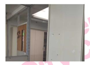
The vertical boxing and panel to boxing (insulating board) (Area: Second Floor, Room 14 Office 3) contains asbestos.
