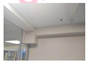
The high level horizontal boxing (insulating board) (Area: Second Floor, Room 19 Finance Office) contains asbestos.
