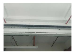
The high level horizontal boxing (insulating board) (Area: Ground Floor, Room 116 Plate Room) contains asbestos.
