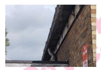
The downpipes to block 1B gable end (Area: Floor 0, Room 152: External) contains asbestos.
