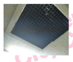
The infill panels – extractor fan housing within ceiling void (insulating board) (Area: Second Floor, Room 31 Bingo Store) contains asbestos.
