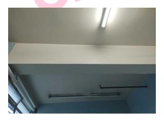
The high level horizontal boxing (insulating board) (Area: Ground Floor, Room 105 Female WC and Lobby) contains asbestos.
