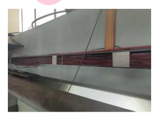
The loose panels within conduits (used as fascia screw panels) (insulating board) (Area: Second Floor, Room 75 Main Workshop) contains asbestos.
