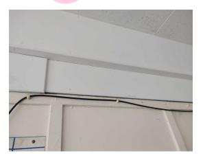
The walls – firebreak panels between RSJ and walls (insulating board) (Area: Second Floor, Room 68 Electric Office) contains asbestos.
