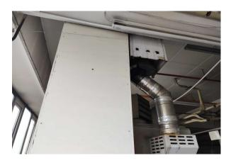
The boxing to heater flue (insulating board) (Area: First Floor, Room 95 Main Printer Workshop) contains asbestos.
