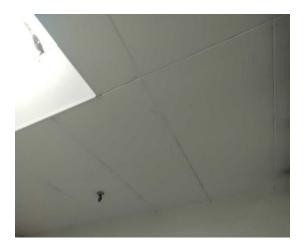
The ceiling tiles (insulating board) (Area: Second Floor, Room 63 Fire Exit Stairwell 3) contains asbestos.
