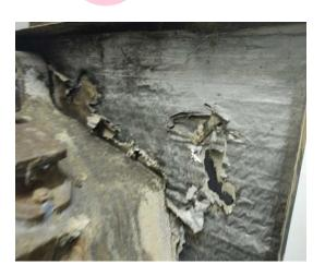
The vessels – aircell lining to boiler (textile) (Area: Second Floor, Room 71 Boiler Room) contains asbestos.
