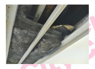
The ceiling (bitumen) (Area: Second Floor, Room 44 Corridor 4) does not contain asbestos.
