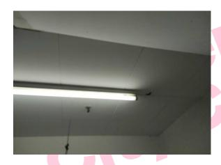
The ceiling tiles (insulating board) (Area: Second Floor, Room 74 Uniform Store) contains asbestos.
