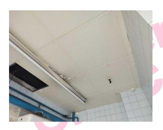
The ceiling tiles (insulating board) (Area: Second Floor, Room 52 Male WC and Lobby) contains asbestos.
