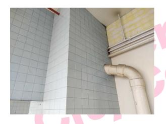
The infill panels – lining to vertical boxing housing flue (insulating board) (Area: First Floor, Room 86 Female WC and Lobby) contains asbestos.
