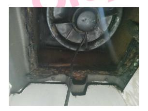
The ceiling – felt to roof (bitumen) (Area: Second Floor, Room 15 Office 4) does not contain asbestos.
