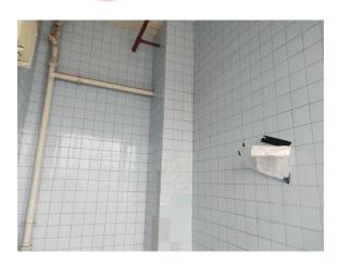
The infill panels – lining to vertical boxing pipework (insulating board) (Area: First Floor, Room 87 Male WC and Lobby) contains asbestos.
