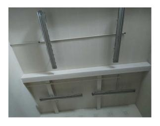
The boxing to high level beams (insulating board) (Area: First Floor, Room 81 Squash Court) contains asbestos.
