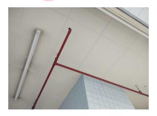
The ceiling (insulating board) (Area: First Floor, Room 87 Male WC and Lobby) contains asbestos.
