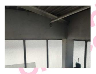
The cladding to RSJ's above and below windows (insulating Board) (Area: Mezzanine Floor, Room 27a: above room 27) contains asbestos.
