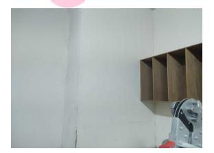
The vertical boxing (insulating board) (Area: Second Floor, Room 6 IT Dept Store) contains asbestos.
