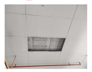
The ceiling (insulating board) (Area: First Floor, Room 84 Maintenance Workshop) contains asbestos.
