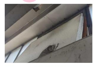
The boxing to RSJ's (insulating Board) (Area: Second Floor, Room 26a: Tank room (within ceiling void)) contains asbestos.
