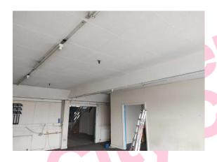
The high level horizontal boxing (insulating board) (Area: Second Floor, Room 68 Electric Office) contains asbestos.
