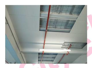
The ceiling (insulating board) (Area: First Floor, Room 90 Print Room) contains asbestos.
