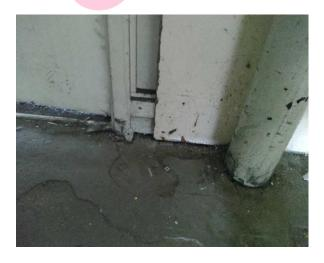
The debris to floor adjacent Electric Office (insulating board) (Area: Second Floor, Room 75 Main Workshop) contains asbestos.
