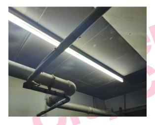
The ceiling tiles (insulating board) (Area: Second Floor, Room 72 Tank Cupboard) contains asbestos.
