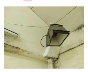
The high level horizontal boxing (insulating board) (Area: Second Floor, Room 74 Uniform Store) contains asbestos.
