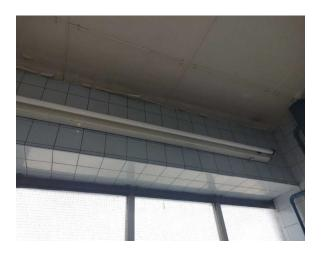
The high level horizontal boxing (insulating board) (Area: Second Floor, Room 52 Male WC and Lobby) contains asbestos.
