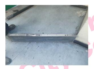
The floor – stair nosing (composite) (Area: Ground Floor, Room 112 Fire Exit Lobby) contains asbestos.
