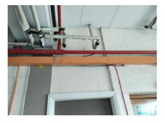
The infill panels – door header above store (79) (insulating board) (Area: First Floor, Room 95 Main Printer Workshop) contains asbestos.
