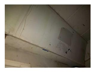
The high level horizontal boxing (insulating board) (Area: Second Floor, Room 73 Paint Store) contains asbestos.
