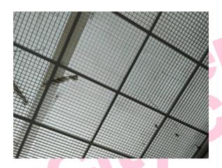
The ceiling tiles (insulating board) (Area: Second Floor, Room 60 Store Room) contains asbestos.
