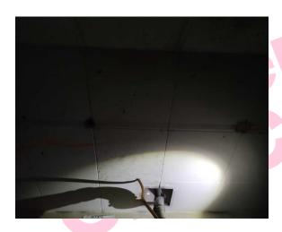
The ceiling tiles (insulating board) (Area: Second Floor, Room 73 Paint Store) contains asbestos.
