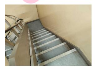
The floor - stair nosings (composite) (Area: Second Floor, Room 5A Fire Exit Stairwell 4) contains asbestos.
