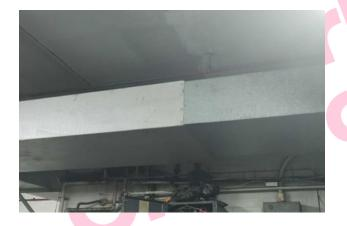
The mastic to the ductwork (Area: Ground Floor, Room 129: Vehicle Maintenance Area) does not contain asbestos.
