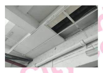
The high level bulkhead boxing (insulating board) (Area: Ground Floor, Room 127: Vehicle Bay 3) contains asbestos.
