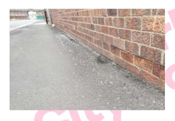
The damp proof course to Block 1A (Area: Floor 0, Room 152: External) contains asbestos.
