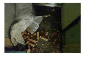
The floor tiles and adhesive (Area: Ground Floor, Room 146: Store Cupboard) contains asbestos.
