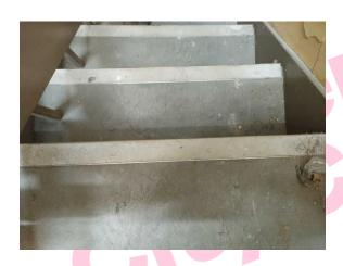
The floor – stair nosings (composite) (Area: First Floor, Room 83 Stairwell) contains asbestos.
