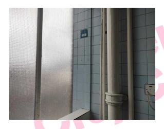
The vertical boxing (behind ceramic tiles) (insulating board) (Area: First Floor, Room 87 Male WC and Lobby) contains asbestos.
