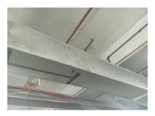
The sealing mastic to ducting joints (mastic) (Area: Ground Floor, Room 119 Main Factory Floor) contains asbestos.
