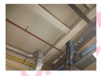
The high level horizontal boxing (insulating board) (Area: Ground Floor, Room 110 Gas Intake / Heater Area) contains asbestos.
