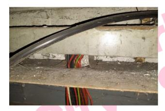
The flashpad used as packer within cable trunking (Area: Ground Floor, Room 131 Vehicle Bay 4 (Unit B)) contains asbestos.
