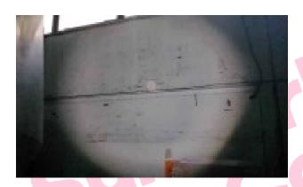
The fascia panels smoke head attached to asbestos (Second Floor Print Room 2/002) are presumed to contain asbestos.
