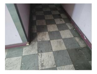
The floor (tiles & adhesive) (Area: Second Floor, Room 61 Corridor and Lift Lobby) does not contain asbestos.
