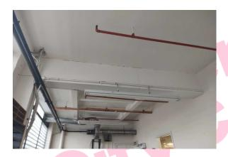
The high level horizontal boxing (insulating board) (Area: Ground Floor, Room 104 Electric Store Room) contains asbestos.
