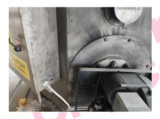
The vessels – gasket to boiler (textile) (Area: First Floor, Room 95 Main Printer Workshop) contains asbestos.
