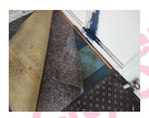
The floor (tiles & adhesive) (Area: Second Floor, Room 68 Electric Office) does not contain asbestos.
