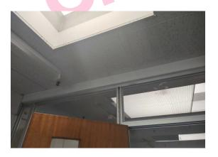
The high level horizontal boxing (insulating board) (Area: Second Floor, Room 15 Office 4) contains asbestos.
