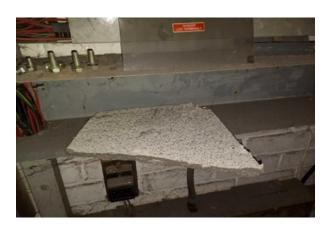
The loose board sittings in trunking (Insulating board) (Area: Ground Floor, Room 131 Vehicle Bay 4 (Unit B)) does not contain asbestos.
