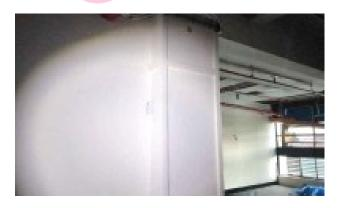
The column cladding inner cladding to column at location of PIR sensor (First Floor Staircase/Stairwell 1/002) is presumed to contain asbestos.
