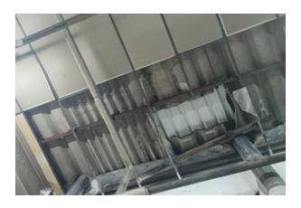
The original roof below new external metal roof (Area: Ground Floor, Room 131 Vehicle Bay 4 (Unit B)) contains asbestos.
