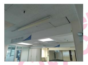
The high level horizontal boxing (insulating board) (Area: Second Floor, Room 26 Main Office) contains asbestos.
