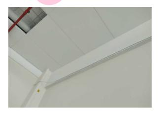
The high level horizontal boxing (insulating board) (Area: First Floor, Room 91 Design Room) contains asbestos.
