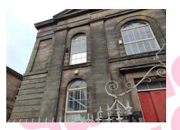
The window - putty to glazing, Area: 38 (External) does not contain asbestos.
