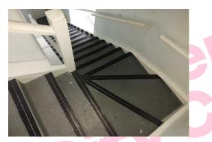
The floor – stair nosing, Area: 1 (Landing and Stairs) does not contain asbestos.
