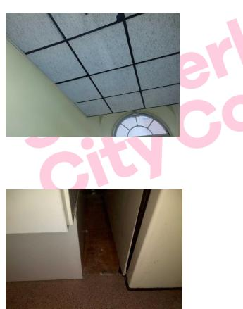
The ceiling - suspended ceiling tiles, Area: 28 (Rear corridor) does not contain asbestos.
