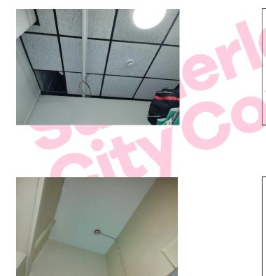
The ceiling - suspended ceiling tiles, Area: 36 (Store cupboard 2) does not contain asbestos.
