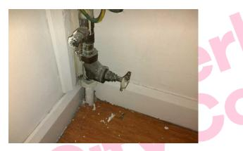
The pipes - gasket to stop tap, Area: 8 (Female wc & lobby) do not contain asbestos.
