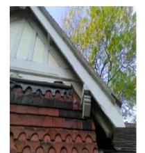
The verge tiles and the cement sheet to the external do not contain asbestos.
