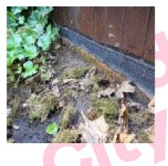
The felt covering to roof external does not contain asbestos.
