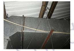
The ceiling – debris to the rear of suspended ceiling tiles & metal ducting (cement) in Area 3 ceiling void 1 contains asbestos.
