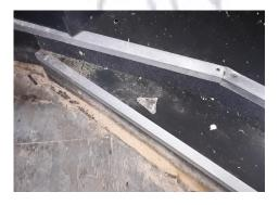
The floor – floor debris (cement) in Area 4 main nightclub & dance floor area contains asbestos.
