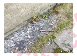
The bitumen felt to floor (External) does not contain asbestos.
