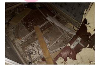
The floor tiles and adhesive (WC) contain asbestos.
