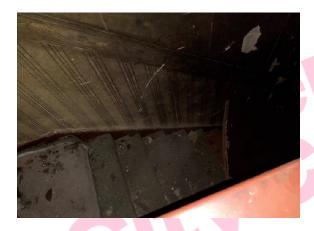
The textured coated ceiling (Stairs and Landing) does not contain asbestos.
