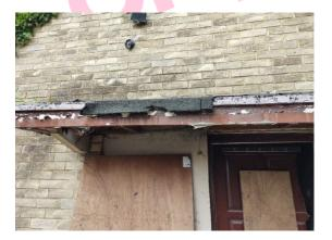
The felt bitumen to canopy roof (External) does not contain asbestos.
