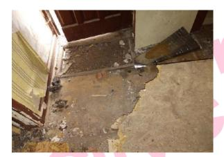
The debris from ceiling to floor (Hall) does not contain asbestos.
