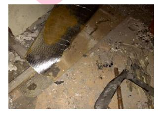
The floor tiles and adhesive (Hall) contain asbestos.
