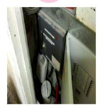
The flash guards within the electrics to the electrical cupboard are presumed to contain asbestos. Any change in its appearance should be noted and passed to Property Services.
