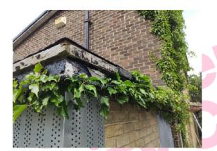
The felt bitumen to outhouse roof (External) does not contain asbestos.
