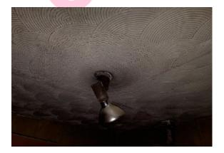
The textured coated ceiling (Bathroom) does not contain asbestos.
