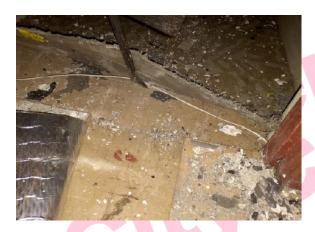
The floor tiles and adhesive (Cupboard Understairs) contain asbestos.
