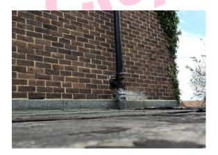
The insulation joint compound to soil pipe (External) contains asbestos.
