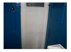
The cement panels to side of door on stairs 2 to second floor and landing does contain asbestos. Any change in its appearance should be recorded, and passed to Property Services.
