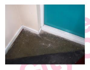
The green vinyl flooring under carpet & adhesive in dressing room 2 does not contain asbestos.
