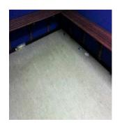
The lino to the Room 3 (Room 10) does not contain asbestos.
