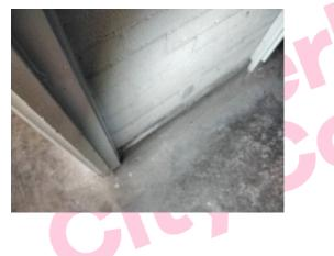
The debris/residue – from deteriorating walls in the toilets including passage (Football Pavilion – G/008) does not contain asbestos.
