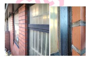
The window putty/seal – frames to wall (External) (Guard House – E/001) contains asbestos.
