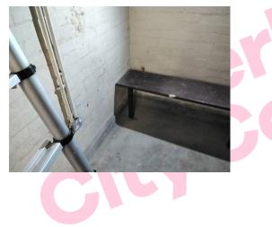
The debris/residue – paint coating from deteriorating walls to floor in the changing room (Football Pavilion – G/010) does not contain asbestos.
