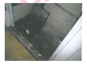
The flooring to Landing Cupboard B (Room 15) does not contain asbestos.
