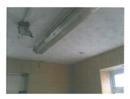
The textured coating to the ceiling in the kitchen (Room 6) does not contain asbestos.
