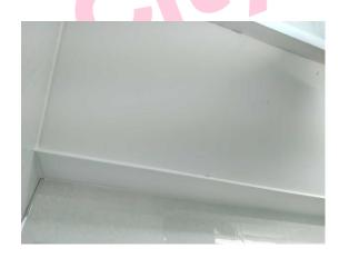
The high level horizontal boxing (insulating board) (Area: Second Floor, Room 17 Female WC and Lobby) contains asbestos.
