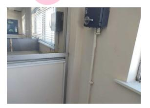
The vertical boxing (insulating board) (Area: Second Floor, Room 4 Store) contains asbestos.
