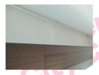
The high level horizontal boxing (insulating board) (Area: Second Floor, Room 35 Paddy Cronin Office) contains asbestos.
