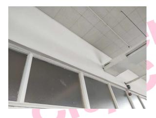
The walls – high level panels (insulating board) (Area: Second Floor, Room 56 Racking Store) contains asbestos.
