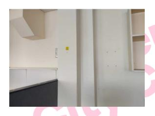
The vertical boxing (insulating board) (Area: Second Floor, Room 5 IT Department) contains asbestos.
