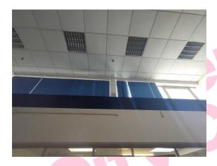
The boxing – cladding to RSJs (insulating board) (Area: Second Floor, Room 18 Contracts Office) contains asbestos.
