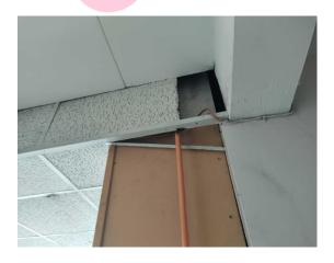
The vertical boxing (insulating board) (Area: Second Floor, Room 61 Corridor and Lift Lobby) contains asbestos.
