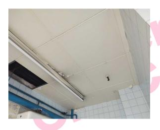
The ceiling tiles (insulating board) (Area: Second Floor, Room 52 Male WC and Lobby) contains asbestos.
