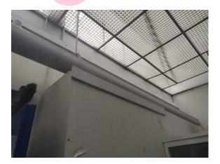
The walls – fillet to top of wall (insulating board) (Area: Second Floor, Room 60 Store Room) contains asbestos.
