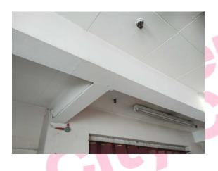
The high level horizontal boxing (insulating board) (Area: Second Floor, Room 61 Corridor and Lift Lobby) contains asbestos.
