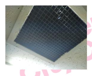
The infill panels – extractor fan housing within ceiling void (insulating board) (Area: Second Floor, Room 31 Bingo Store) contains asbestos.
