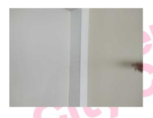
The vertical boxing (insulating board) (Area: Second Floor, Room 28 Canteen) contains asbestos.
