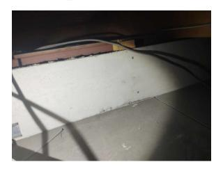
The debris to tops of ceiling tiles (insulating board) (Area: Second Floor, Room 8 Server Room) contains asbestos.
