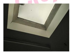
The infill panels – upstands to skylights (insulating board) (Area: Second Floor, Room 16 Male WC and Lobby) contains asbestos.
