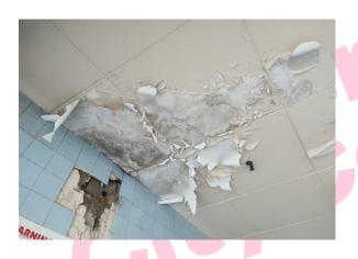
The ceiling tiles (insulating board) (Area: Second Floor, Room 51 Female WC and Lobby 2) contains asbestos.
