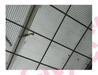
The ceiling tiles (insulating board) (Area: Second Floor, Room 60 Store Room) contains asbestos.
