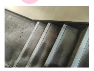
The floor – stair nosings (composite) (Area: Second Floor, Room 46 Fire Exit Stairwell 1) contains asbestos.
