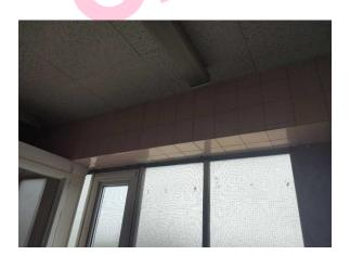
The high level horizontal boxing (insulating board) (Area: Second Floor, Room 48 First Aid Room) contains asbestos.
