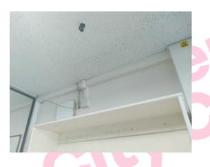
The high level horizontal boxing (insulating board) (Area: Second Floor, Room 21 Office 6) contains asbestos.
