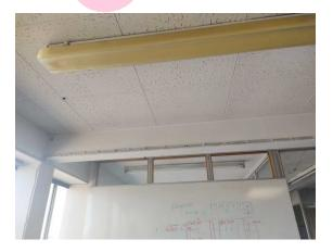
The high level horizontal boxing (insulating board) (Area: Second Floor, Room 10 EPS Department) contains asbestos.
