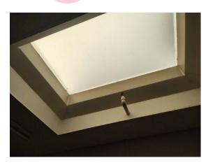
The infill panels – upstands to skylight (insulating board) (Area: Second Floor, Room 26 Main Office) contains asbestos.
