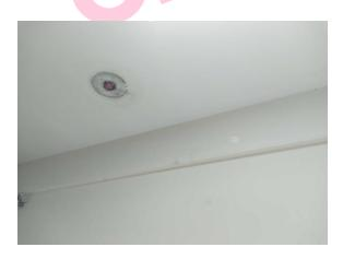
The high level horizontal boxing (insulating board) (Area: Second Floor, Room 45 Key Cupboard) contains asbestos.
