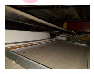
The debris to tops of ceiling tiles (insulating board) (Area: Second Floor, Room 40 Reception) contains asbestos.
