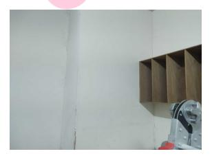
The vertical boxing (insulating board) (Area: Second Floor, Room 6 IT Dept Store) contains asbestos.
