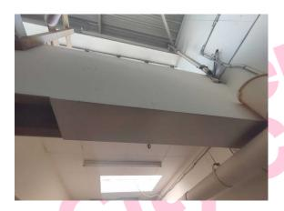
The high level horizontal boxing (insulating board) (Area: Second Floor, Room 27 Store Room) contains asbestos.
