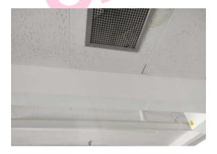
The high level horizontal boxing (insulating board) (Area: Second Floor, Room 14 Office 3) contains asbestos.
