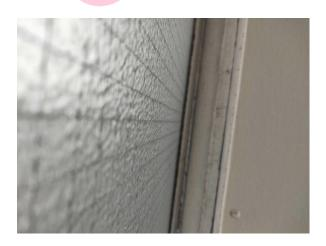
The window – fillet to window reveal behind cladded RSJ (insulating board) (Area: Second Floor, Room 47 Comms Room) contains asbestos.
