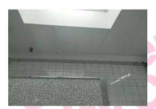
The high level horizontal boxing (insulating board) (Area: Second Floor, Room 16 Male WC and Lobby) contains asbestos.
