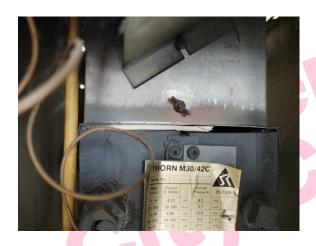
The vessels – lining to boiler (millboard) (Area: Second Floor, Room 56 Racking Store) contains asbestos.
