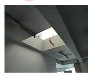
The infill panels – upstands to skylights (insulating board) (Area: Second Floor, Room 61 Corridor and Lift Lobby) contains asbestos.
