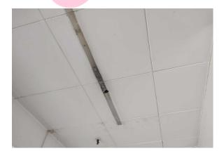
The ceiling tiles (insulating board) (Area: Second Floor, Room 50 Corridor 6) contains asbestos.
