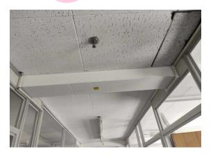
The high level horizontal boxing (insulating board) (Area: Second Floor, Room 7 Corridor) contains asbestos.
