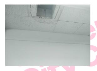
The walls – firebreak above door (insulating board) (Area: Second Floor, Room 15 Office 4) contains asbestos.
