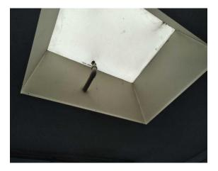
The infill panels – upstands to skylights (insulating board) (Area: Second Floor, Room 56 Racking Store) contains asbestos.
