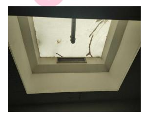
The infill panels – upstands to skylight (insulating board) (Area: Second Floor, Room 37 Corridor 3) contains asbestos.
