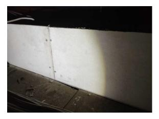
The debris to tops of ceiling tiles (insulating board) (Area: Second Floor, Room 1 Meeting Room) contains asbestos.
