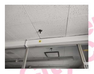
The high level horizontal boxing (insulating board) (Area: Second Floor, Room 4 Store) contains asbestos.
