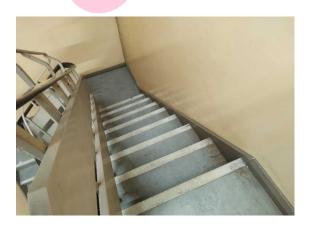
The floor - stair nosings (composite) (Area: Second Floor, Room 5A Fire Exit Stairwell 4) contains asbestos.
