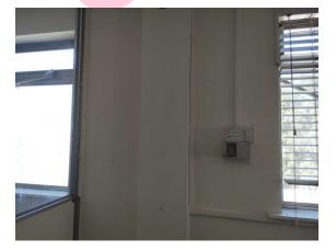
The vertical boxing (insulating board) (Area: Second Floor, Room 3 Office 2) contains asbestos.
