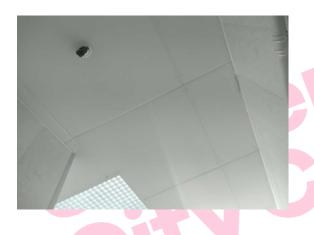
The ceiling tiles (insulating board) (Area: Second Floor, Room 17 Female WC and Lobby) contains asbestos.
