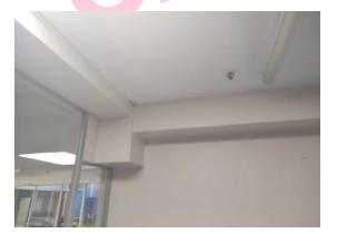
The high level horizontal boxing (insulating board) (Area: Second Floor, Room 19 Finance Office) contains asbestos.
