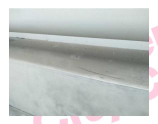
The fillet to top of wall (insulating board) (Area: Second Floor, Room 60 Store Room) contains asbestos.
