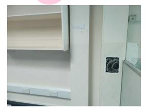
The vertical boxing (insulating board) (Area: Second Floor, Room 21 Office 6) contains asbestos.
