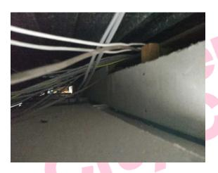
The debris to tops of ceiling tiles (insulating board) (Area: Second Floor, Room 1 Meeting Room) contains asbestos.
