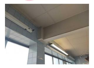
The high level horizontal boxing (insulating board) (Area: Second Floor, Room 51 Female WC and Lobby 2) contains asbestos.
