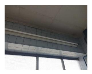
The high level horizontal boxing (insulating board) (Area: Second Floor, Room 52 Male WC and Lobby) contains asbestos.
