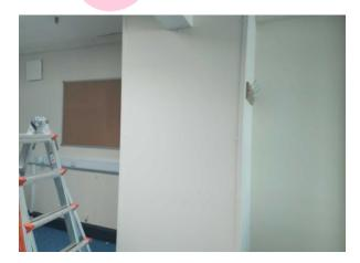
The vertical boxing behind wood cladding (insulating board) (Area: Second Floor, Room 20 Office 5) contains asbestos.
