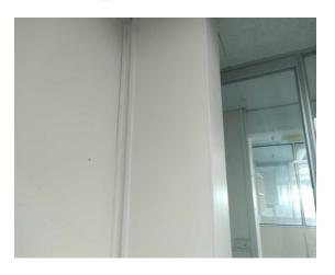
The vertical boxing (insulating board) (Area: Second Floor, Room 23 Office 8) contains asbestos.
