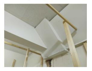
The high level horizontal boxing (insulating board) (Area: Second Floor, Room 31 Bingo Store) contains asbestos.
