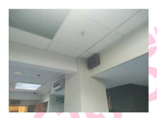
The high level horizontal boxing (insulating board) (Area: Second Floor, Room 40 Reception) contains asbestos.
