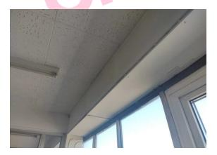
The vertical boxing (insulating board) (Area: Second Floor, Room 13 Petty Cash Office) contains asbestos.
