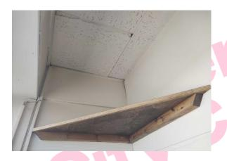
The walls – firebreak above door (insulating board) (Area: Second Floor, Room 13 Petty Cash Office) contains asbestos.
