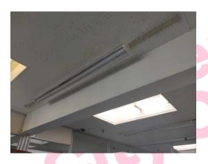
The high level horizontal boxing (insulating board) (Area: Second Floor, Room 20 Office 5) contains asbestos.
