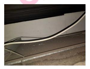
The debris to tops of ceiling tiles (insulating board) (Area: Second Floor, Room 19 Finance Office) contains asbestos.
