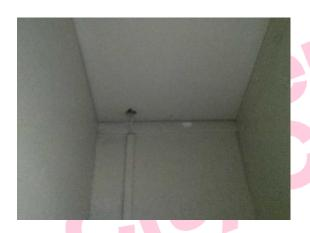
The walls – firebreak to top of wall (insulating board) (Area: Second Floor, Room 41 Cupboard) contains asbestos.
