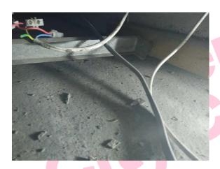
The debris to tops of ceiling tiles (insulating board) (Area: Second Floor, Room 6 IT Dept Store) contains asbestos.
