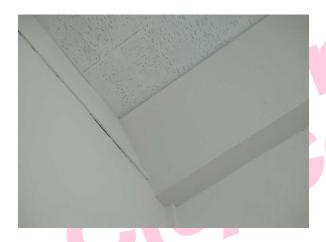
The high level horizontal boxing (insulating board) (Area: Second Floor, Room 54 Ex Store) contains asbestos.
