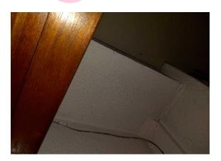
The high level horizontal boxing (insulating board) (Area: Second Floor, Room 42 Sound Cupboard) contains asbestos.
