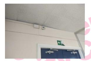
The walls – firebreak above door (insulating board) (Area: Second Floor, Room 11 Corridor) contains asbestos.
