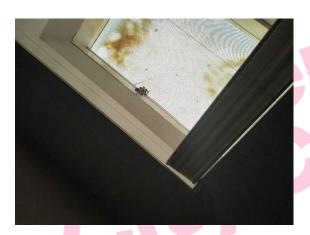
The infill panels – upstands to skylight (insulating board) (Area: Second Floor, Room 25 Finance Room 2) contains asbestos.
