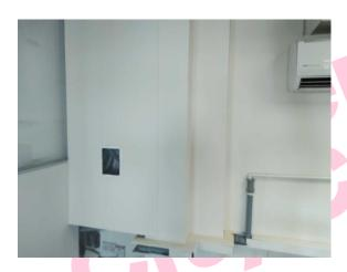
The vertical boxing (insulating board) (Area: Second Floor, Room 8 Server Room) contains asbestos.
