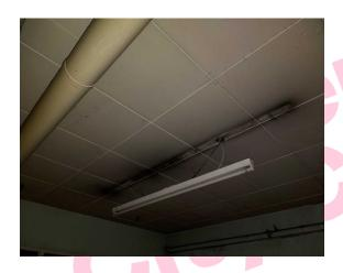
The ceiling tiles (insulating board) (Area: Second Floor, Room 61 Corridor and Lift Lobby) contains asbestos.
