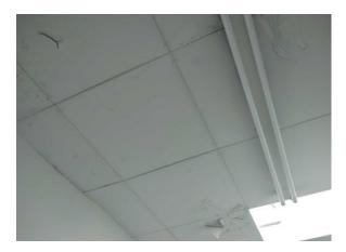
The ceiling tiles (insulating board) (Area: Second Floor, Room 49 Corridor 5) contains asbestos.
