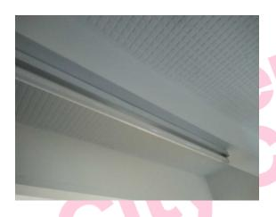
The high level horizontal boxing (insulating board) (Area: Second Floor, Room 37 Corridor 3) contains asbestos.
