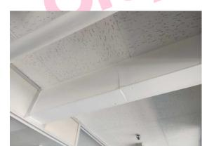
The high level horizontal boxing (insulating board) (Area: Second Floor, Room 11 Corridor) contains asbestos.
