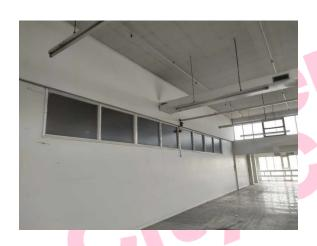
The window – beading to high level windows (insulating board) (Area: Second Floor, Room 56 Racking Store) contains asbestos.
