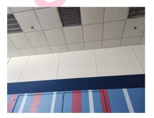
The walls – panels to high level wall (insulating board) (Area: Second Floor, Room 18 Contracts Office) contains asbestos.
