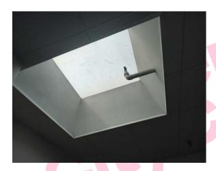
The infill panels – upstands to skylights (insulating board) (Area: Second Floor, Room 46 Fire Exit Stairwell 1) contains asbestos.
