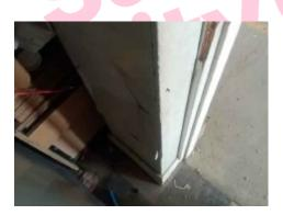
The boxing vertical damaged (enclose or removal required) in First Floor Cupboard Store Room 1/078 contains asbestos.
