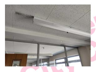
The high level horizontal boxing (insulating board) (Area: Second Floor, Room 3 Office 2) contains asbestos.
