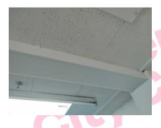
The high level horizontal boxing behind wood cladding (insulating board) (Area: Second Floor, Room 9 Sales Office) contains asbestos.
