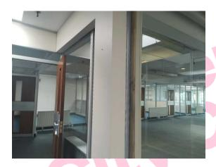
The vertical boxing (insulating board) (Area: Second Floor, Room 19 Finance Office) contains asbestos.
