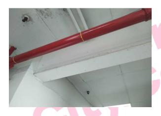
The high level horizontal boxing (insulating board) (Area: Second Floor, Room 49 Corridor 5) contains asbestos.
