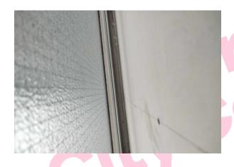
The window – fillet to window reveal behind cladded RSJ (insulating board) (Area: Second Floor, Room 48 First Aid Room) contains asbestos.
