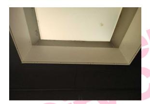
The infill panels – upstands to skylight (insulating board) (Area: Second Floor, Room 10 EPS Department) contains asbestos.
