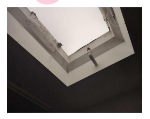
The infill panels – upstands to skylight (insulating board) (Area: Second Floor, Room 27 Store Room) contains asbestos.
