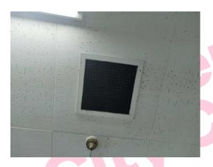
The infill panels – extractor fan housing within ceiling void (insulating board) (Area: Second Floor, Room 32 Prom Games Store) contains asbestos.
