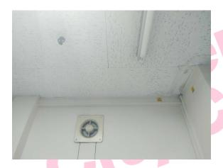
The high level horizontal boxing (insulating board) (Area: Second Floor, Room 23 Office 8) contains asbestos.
