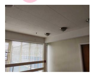
The high level horizontal boxing (insulating board) (Area: Second Floor, Room 58 Private Dining Room) contains asbestos.
