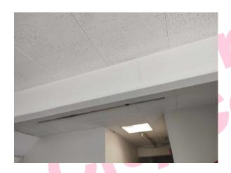
The high level horizontal boxing (insulating board) (Area: Second Floor, Room 50 Corridor 6) contains asbestos.
