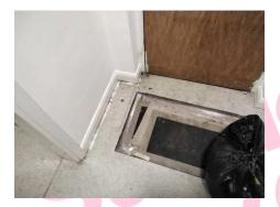
The Floor - adhesive residue – bitumen in Tea Rooms G/006 Passageway contains asbestos.
