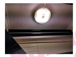
The Ceiling - Insulating Board in Boiler House/Changing Rooms G/017 Toilets contains asbestos.
