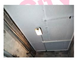
The Ceiling - Insulating Board in Boiler House/Changing Rooms G/007 Cupboard-Store contains asbestos.
