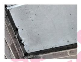
The Ceiling - Insulating Board in Boiler House/Changing Rooms G/006 Passageway contains asbestos.
