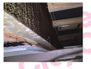
The debris within nail holes (Toilets G/011) (Older Building – The Oval) contains asbestos.
