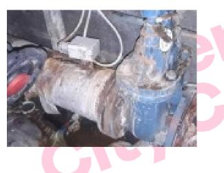
The pipework gasket to bottom pipework V28 left side (Boiler Room G/001 – The Oval) does contain asbestos.
