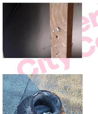
The minor sporadic residue to existing nails in the ceiling (Area 2/Annexe room ceiling void) does contain asbestos.
