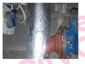
The pipework gasket to pipework V12 left side (Boiler Room G/001 – The Oval) does contain asbestos.
