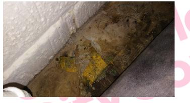
The subfloor in 019/WC contains asbestos.
