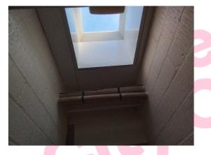
The ceiling (Female Toilets G/019) (Older Building – The Oval) contains asbestos.
