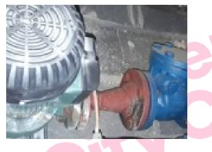
The pipework gasket to pipework V10 right side (Boiler Room G/001 – The Oval) does contain asbestos.
