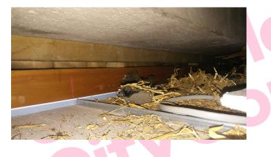
The debris above doors leading to 003 in 001/Entrance lobby void above contains asbestos.
