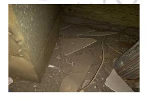
The floor – broken insulating board panels within riser (insulating board) (area: 12a riser) contains asbestos.
