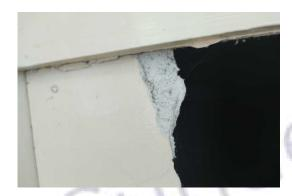
The walls – wall panels to riser 12a (insulating board) (area: 12a riser) contain asbestos.
