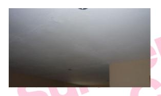
The coating to the ceiling in the living room (Rm 0/03) contains asbestos. Any change in its appearance should be recorded, and passed to Property Services.
