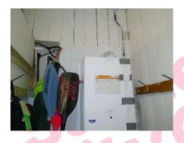
The mounting board to boiler in Watersports store/0/002 does not contain asbestos.
