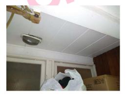
The ceiling in Rear porch 0/010 contains asbestos.
