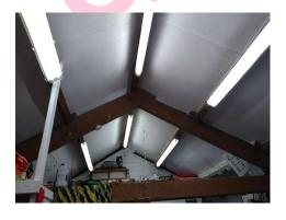
The paper lining to ceiling panels in First floor/1/001 does not contain asbestos.
