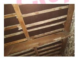
The sarking in Watersports store loft above/0/002 does not contain asbestos.
