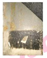
The sub floor covering in Bedroom/0/001 contains asbestos.
