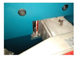
The gasket to boiler front in Boiler Room/-1/002 does not contain asbestos.
