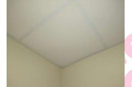
The suspended ceiling in Bedroom 16 ensuite bathroom/0/002 does not contain asbestos.
