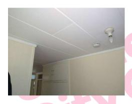
The ceiling in Hallway 0/004 contains asbestos.
