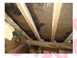
The sarking in First floor/1/001 does not contain asbestos.
