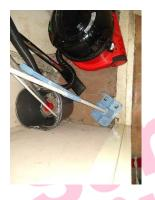
The floor covering in Kitchen cupboard/0/002 contains asbestos.
