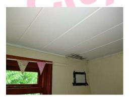
The ceiling in Kitchen/0/002 contains asbestos.
