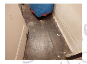
The brown sheet vinyl (Emergency Lighting Room/Area 5) does not contain asbestos.
