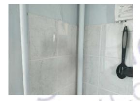
The walls behind ceramic tiles (Kitchen/Area 12) do not contain asbestos.
