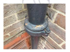
The soil pipe joint capping (External/Area 16) does not contain asbestos.
