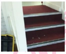
The Floor – stair nosing (bitumen) in Area 1 (Classroom) does not contain asbestos.
