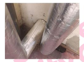
The debris/residue to floor and unlagged pipes Ground Floor, Cupboard, G.001 contains asbestos.
