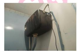
The toilet (Bakelite) contains asbestos.
