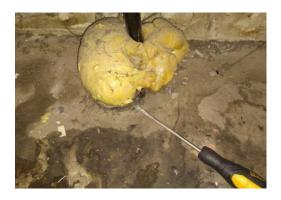
The cable intrusion sleeve (Area 46/Electric meter cupboard) does not contain asbestos.
