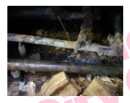
The Debris residue from pipework (Floor duct G/01 Hall KS2) does not contain asbestos.
