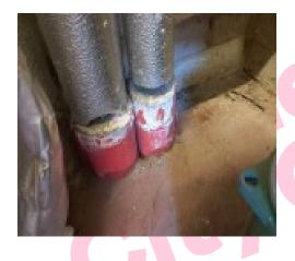
The lagging pipework (Keystage 1 Plant Room G/01) does not contain asbestos.
