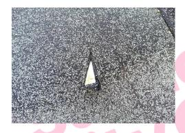
The bitumen roof felt (Area 1/External) does not contain asbestos.
