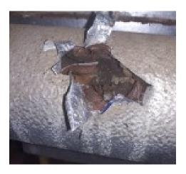
The Paper lining – plant pipework behind metal casing (Keystage 1 Plant Room G/01)does not contain asbestos.
