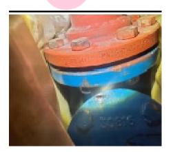
The - Gaskets pipework at high level and behind plant RHS side (Keystage 1 Plant Room G/01) does not contain asbestos.
