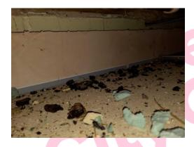
The ceiling (Area 79/Toilet) does not contain asbestos.
