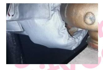
The acoustic pads beneath 2 x pumps (Boiler Room/Area 001) do not contain asbestos.
