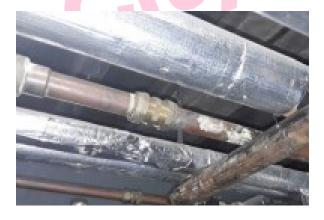
pipework and hangers beneath foam insulation (Boiler Room/Area 001) contains asbestos.
