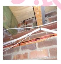
The bitumen overspill - to walls/cabling in void (Nursery G/13) does not contain asbestos.
