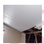
The textured coating - to ceiling (Roof void 4 R/04) does not contain asbestos.
