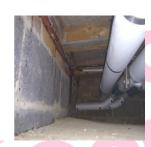
The bitumen overspill - to ceiling void walls (Store G/11) does not contain asbestos.
