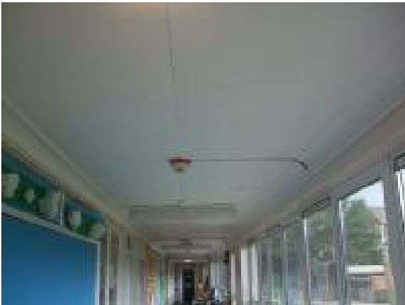
The ceiling board (Corridor 4/060) does not contain asbestos.
