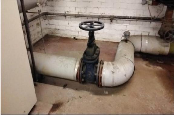
The pipework gaskets return flow valve and end stop in the Boiler Room Z/001 does not contain asbestos.
