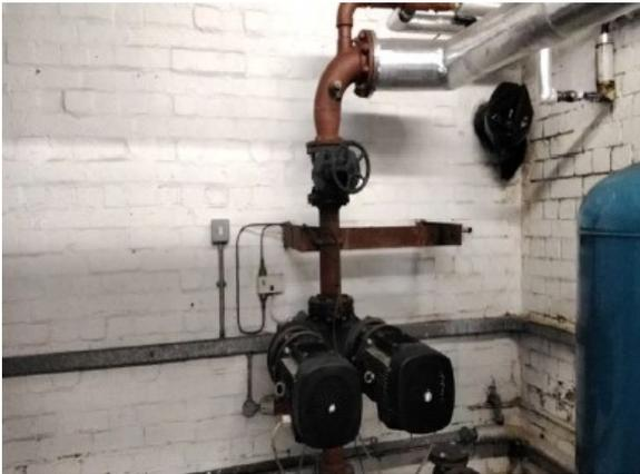
The pipework gaskets grunfos pumps in the Boiler Room Z/001 does not contain asbestos.
