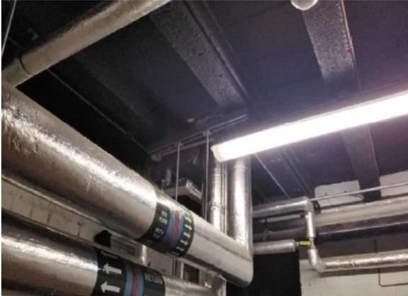
The debris/residue to the ceiling in the Boiler Room Z/001 does not contain asbestos.
