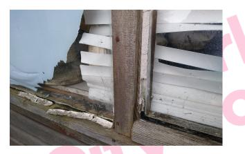
The putty to glazing in the caretaker's house (External) does not contain asbestos.
