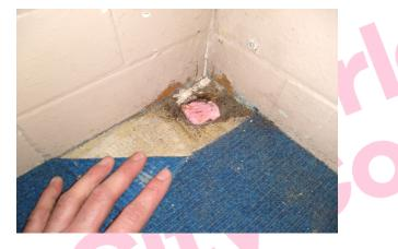
The subfloor to mezzanine in the stairwell landing (Rm 1/09) does not contain asbestos.
