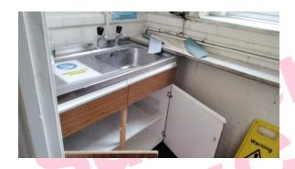
The Pipework to sink wate pipe (Corridor 1/019) does not contain asbestos.
