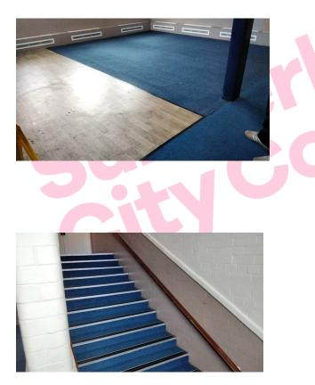
The Floor adhesive (Landing MZ/003) contains asbestos.
