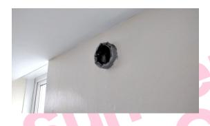
The Flue Pipe (Corridor G/010) contains asbestos.
