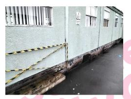
The wall coating (External/E002) does not contain asbestos.
