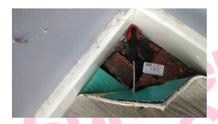
The Floor tile red thicker/older type (Corridor G/010) contains asbestos.
