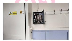
The Electrical Services Fuses/Flashguards (Corridor G/010) contains asbestos.
