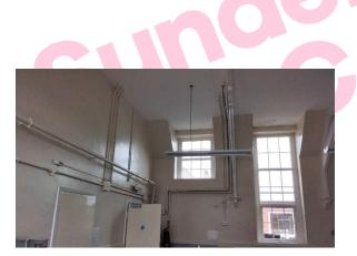
The Ceiling inspected within (Office G/007) does not contain asbestos.
