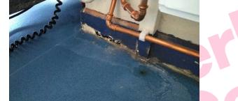
The Floor covering adhesive residue (Kitchen G/006) contains asbestos.
