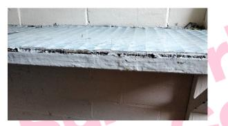
The Shelving heat pads to bottom and underside of shelf above (Cupboard Store G/034) contain asbestos.
