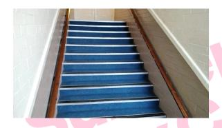
The Floor nosing to stairs (Landing MZ/001) does not contain asbestos.
