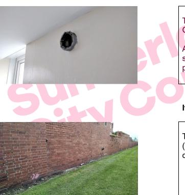
The Flue Pipe (Corridor G/010) contains asbestos.
