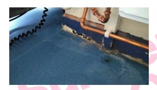
The Floor covering adhesive residue (Kitchen G/006) contains asbestos.
