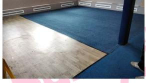
The Floor adhesive (Landing MZ/003) contains asbestos.
