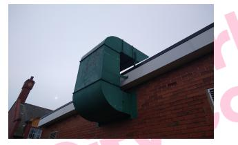
The sealant to extractor ducting joints to the Dining hall building (External) does not contain asbestos.
