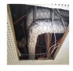
The rope pipework insulation (Classroom 5 G/01) does not contain asbestos.
