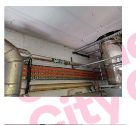
The flat ceiling panels (Rm 0/27 Boiler Room adj Kitchen) contains asbestos.
