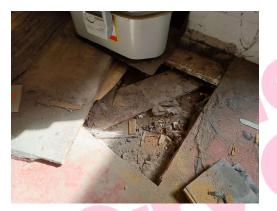
The debris within gas box sump (Rm 0/26 KS1 Boiler Room) does not contain asbestos.
