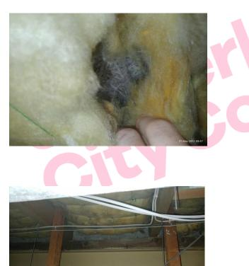
The ceiling (Strawboard) (Lobby G0/27 False ceiling void/Area 2) does not contain asbestos.
