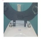
The composite material -Toilet seat (W/C G/44) does not contain asbestos.
