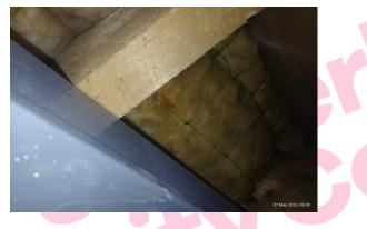
The ceiling (Strawboard) (Classroom 3 G0/23 False ceiling void/Area 4) does not contain asbestos.
