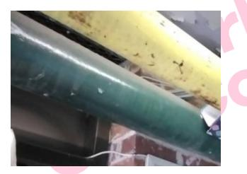
The pipework insulation in the Store Room (G/002) does not contain asbestos.
