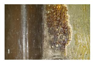
The adhesive backing to lino subfloor to the ramped corridor does contain asbestos.
