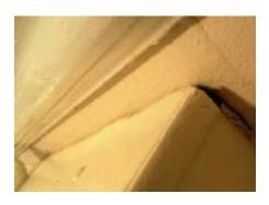
The foam between the metal rad hangers and brick wall in the corridor (Room 35) does not contain asbestos.
