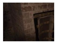
There is possibly asbestos within the sealed brick riser in the plant room (Sub level Room 1). Prior to any intrusive works, a survey must be carried out.
