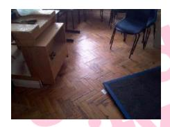
The bitumen beneath the parquet flooring in the joinery Room (Room 40) is presumed to contain asbestos.
