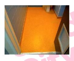
The bitumen beneath the modern lino and the parquet flooring in the community room wc (Room 37) is presumed to contain asbestos.
