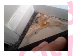
The remaining adhesive to the floor beneath the carpet and modern screed in the repro room (Room 16) contains asbestos.
