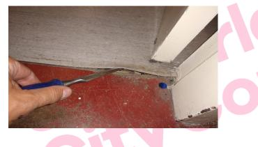
The floor tile with bitumen adhesive in 0/013 Classroom contains asbestos.
