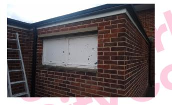
The sealant to metal window frames (External) contains asbestos.
