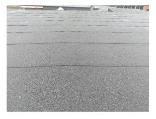
The bitumen lining roof (External E/001) does not contain asbestos.
