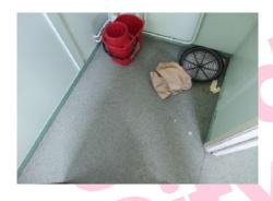
The composite floor (Area 8/Staff WC) does not contain asbestos.
