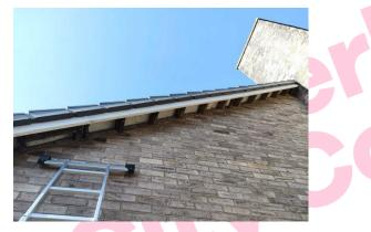
The residue to nails to former gable end soffits of Children's centre (Area 129/External) does not contain asbestos.
