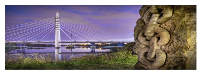
The road bridge is a two-span cable-stayed bridge with an A-frame pylon rising to 105m (344ft) crossing the River Wear between Castletown on the north to Pallion on the south bank.
