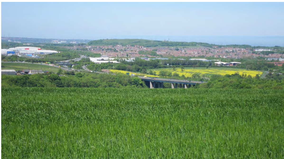
Hylton Bridge, looking towards North Hylton
