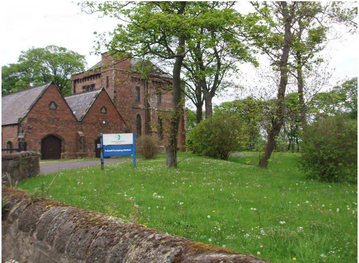
Fulwell Pumping Station (field RE18)
