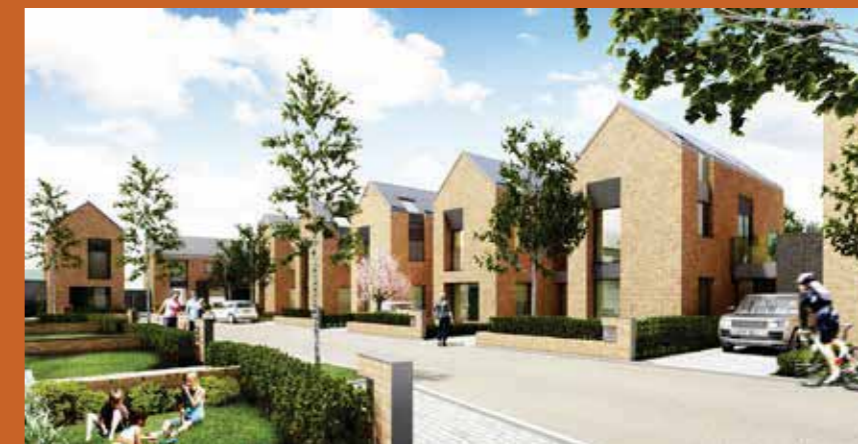
2 storey housing, Musker Street, Crosby. The properties have large front gardens, and trees are planted along the street.
