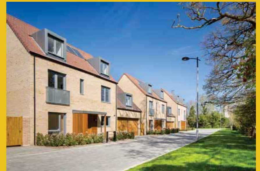
Housing at Trumpington Meadows, Cambridge. The building line is close to the edge of the pavement, creating a strong frontage onto the street.
