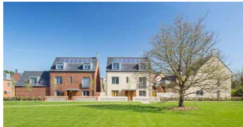
2 storey Barratt Homes at Trumpington Meadows, with dormer windows
