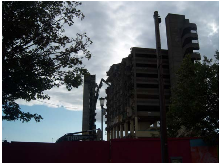
Gateshead car park undergoing demolition
