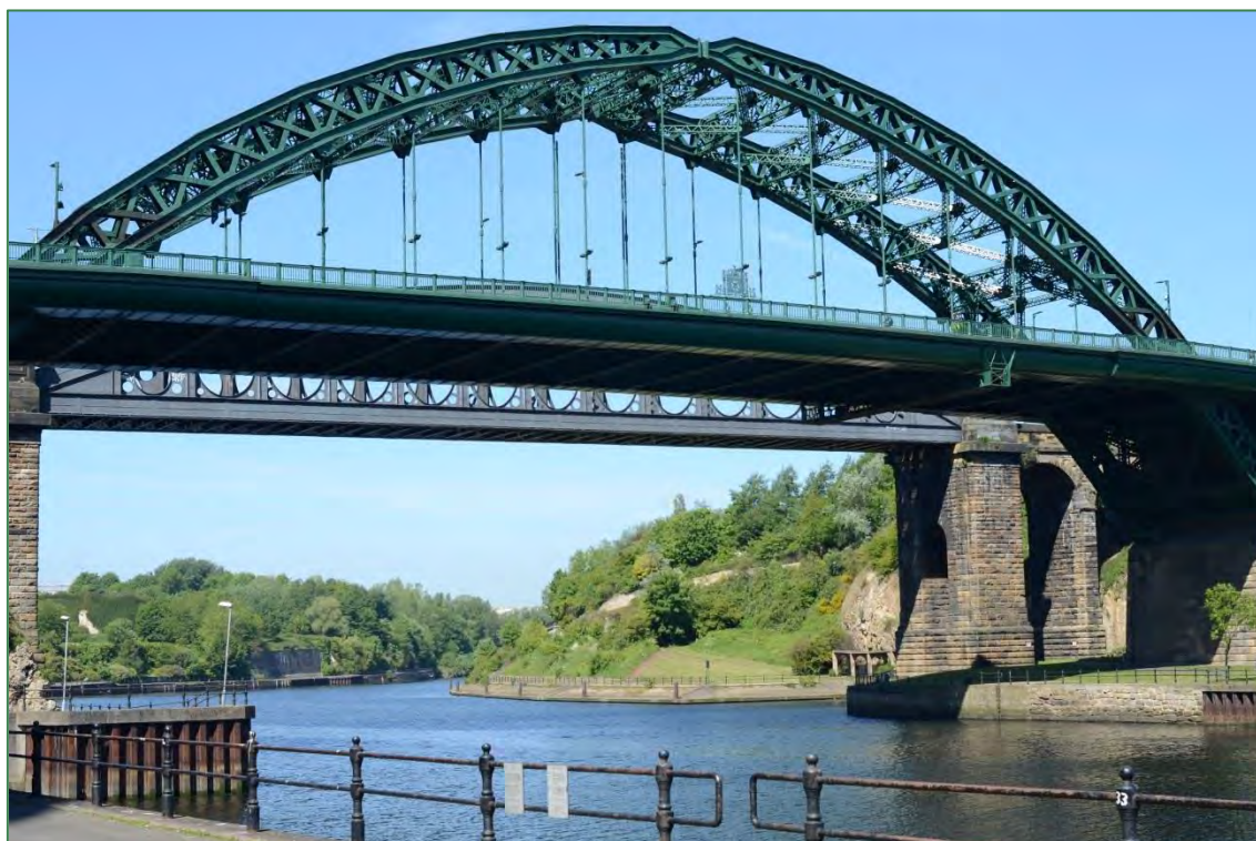
Figure 2.1 The Wearmouth Bridge spans the river gorge at Sunderland
