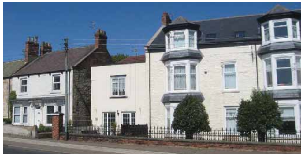
The striking white rendered frontages and features such as bay windows and Welsh slate roofs distinguish the above group of houses; it is important such characteristics are protected from inappropriate alteration or replacement.
