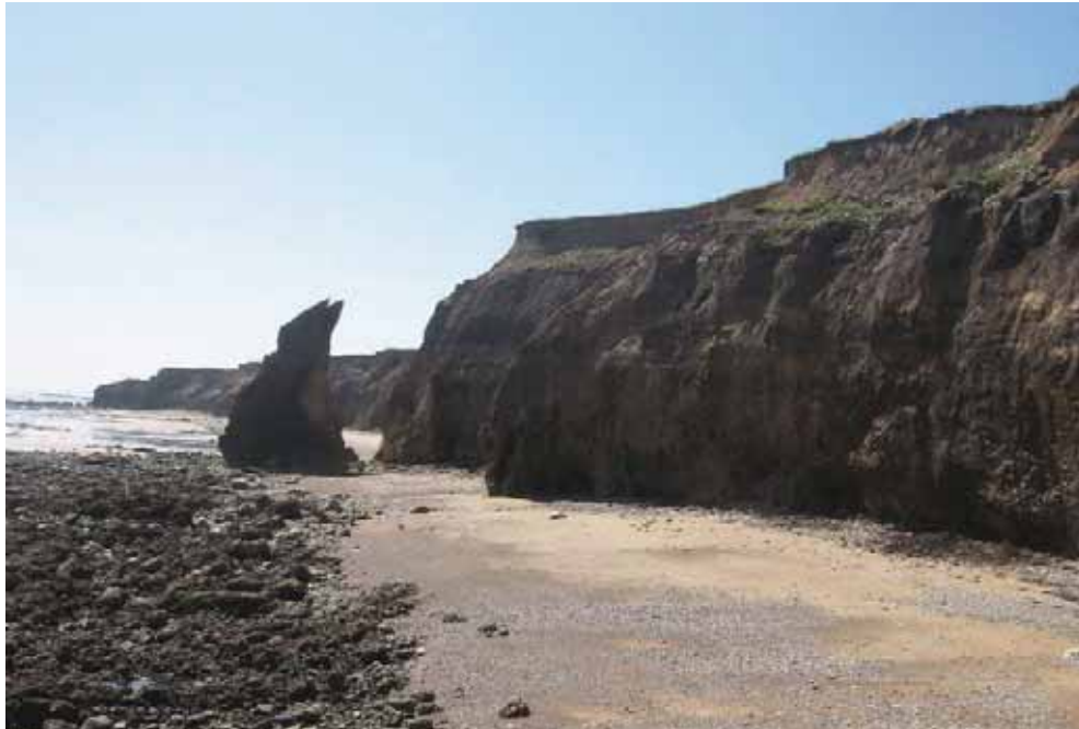
Coastal erosion of the magnesian limestone Ryhope Cliffs, part of the defined Durham Heritage Coast and historically a source of building material for the village
