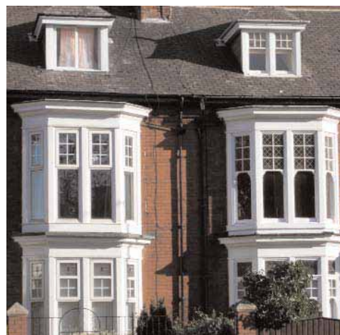
The visual impact of uPVC windows in an otherwise uniform terrace
