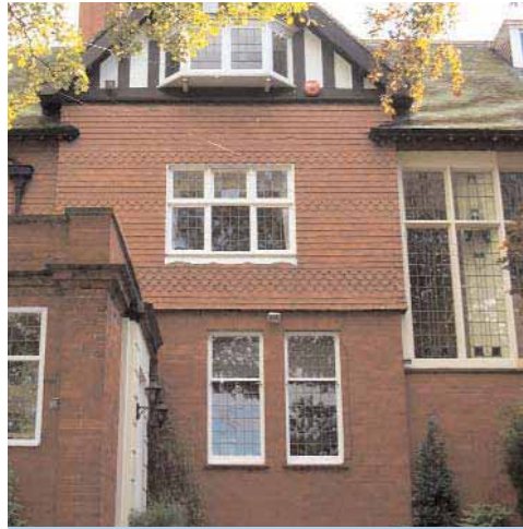
Terracotta tile hung front elevation
