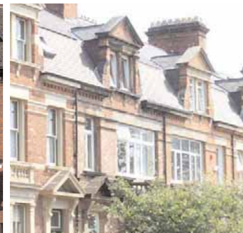
The visual impact of dramatic alterations such as the insertion of picture windows
