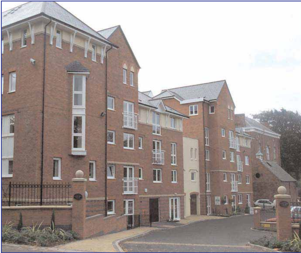
This development has used the steep topography of the site to its advantage whilst also respecting the scale, style and materials of the adjacent Victorian villa.
