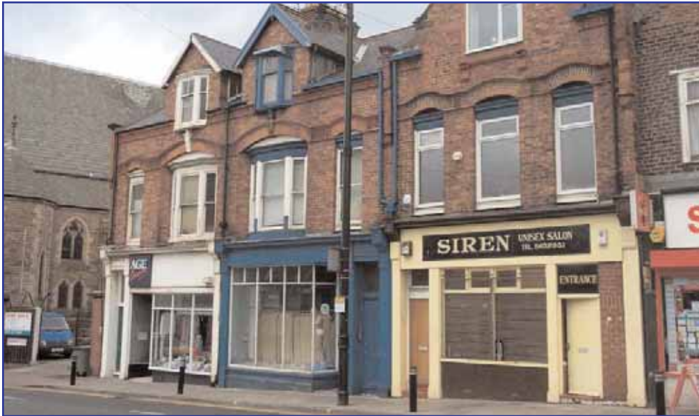
Several buildings along Stockton Road contain retail outlets at street level and have retained many original shopfront features, such as the carved timber pilasters and cornices.
