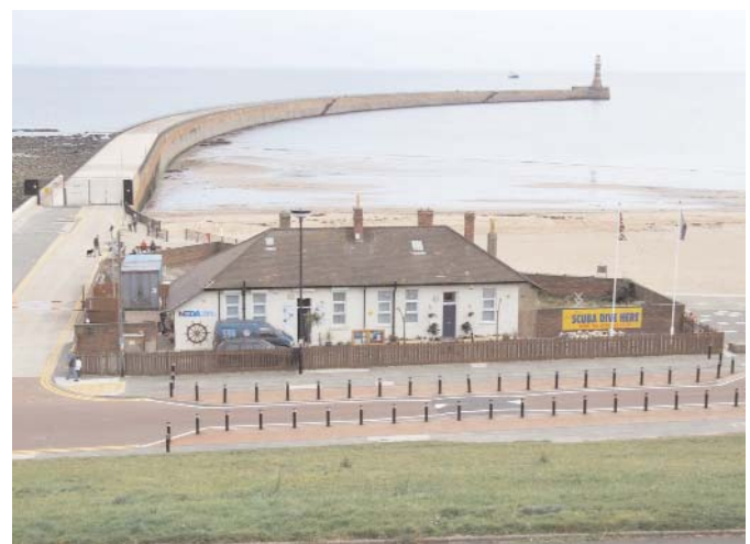
Lighthouse keepers' cottages
