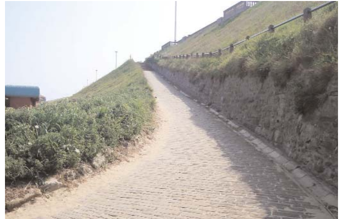
Steep pathways lack handrail
