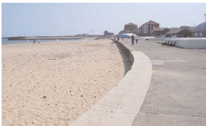
Lack of ramped access to beach
