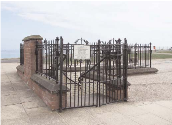
Underground toilets at Seaburn
