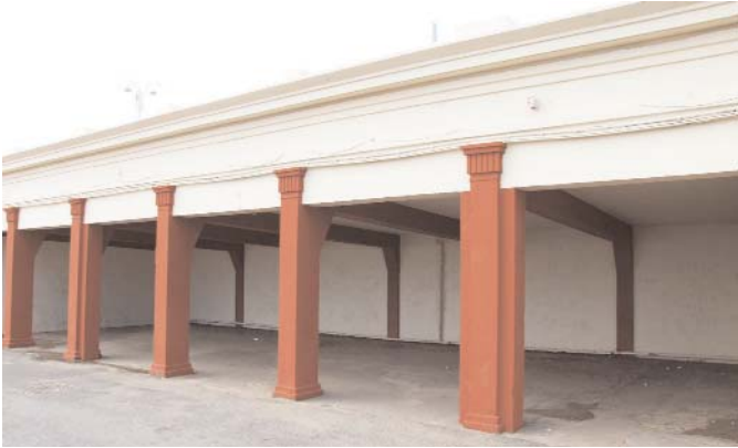
Seating removed from Seaburn shelter due to vandalism
